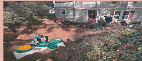
Fuji Clean CEN Series Installation in Sea Cliff, NY - Installation by Discount Cesspool.
