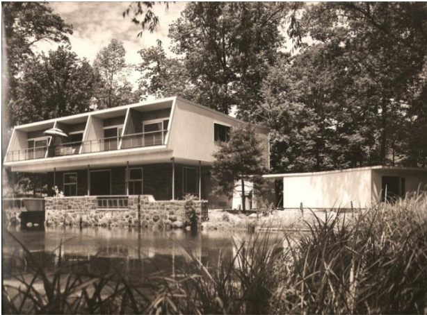
New 2 nd floor on ice house stone walls
