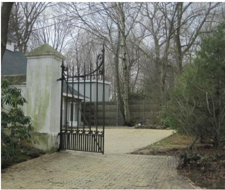
Remaining metal gate and pillar to stable yard
